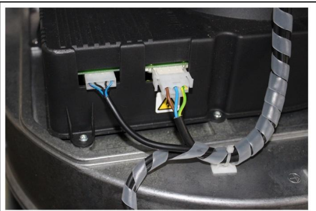
MODULATED FAN CONNECTIONS
